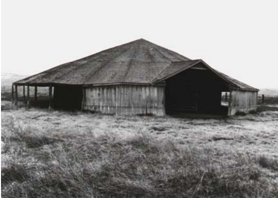
Peter French's Round Barn, constructed in 1870s
